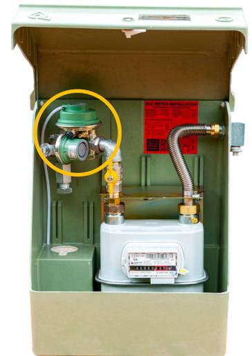
**This regulator is used in all medium pressure meter box assemblies supplied by Clesse UK.**
